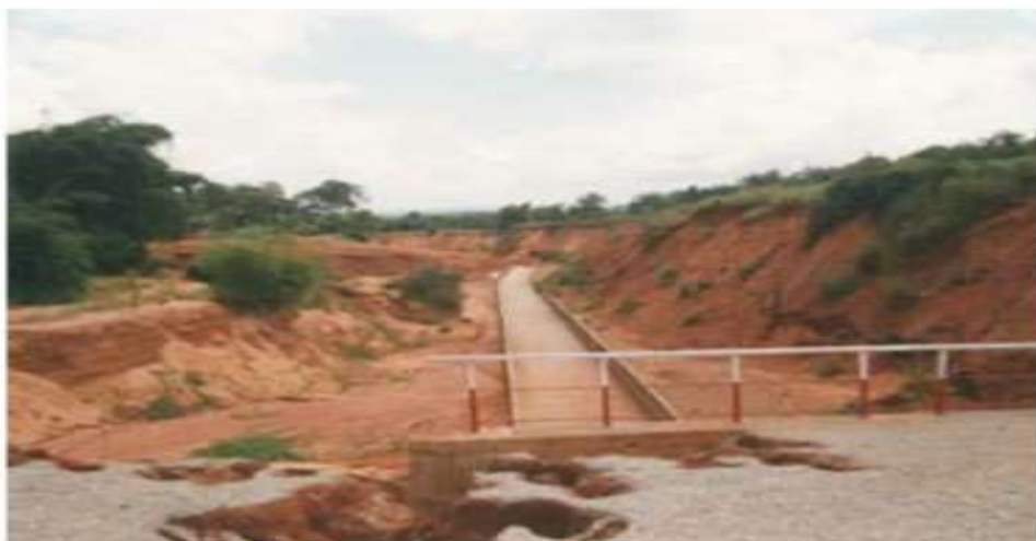
Plate 4 A site in Umuchu Anambra State
