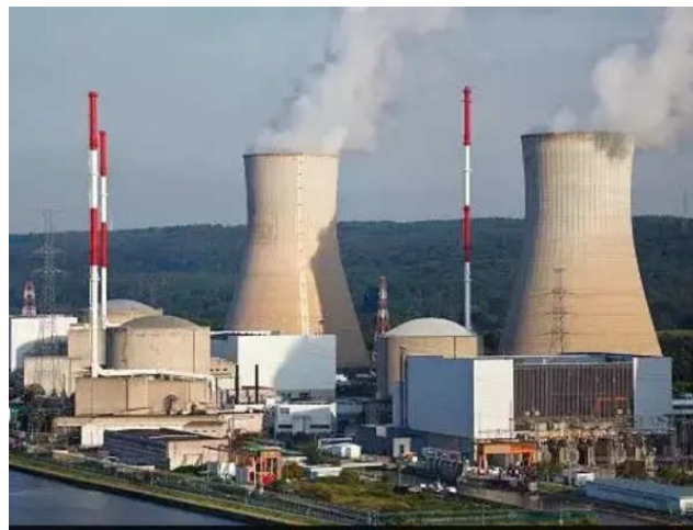
Figure 1: Nuclear Power Plant
