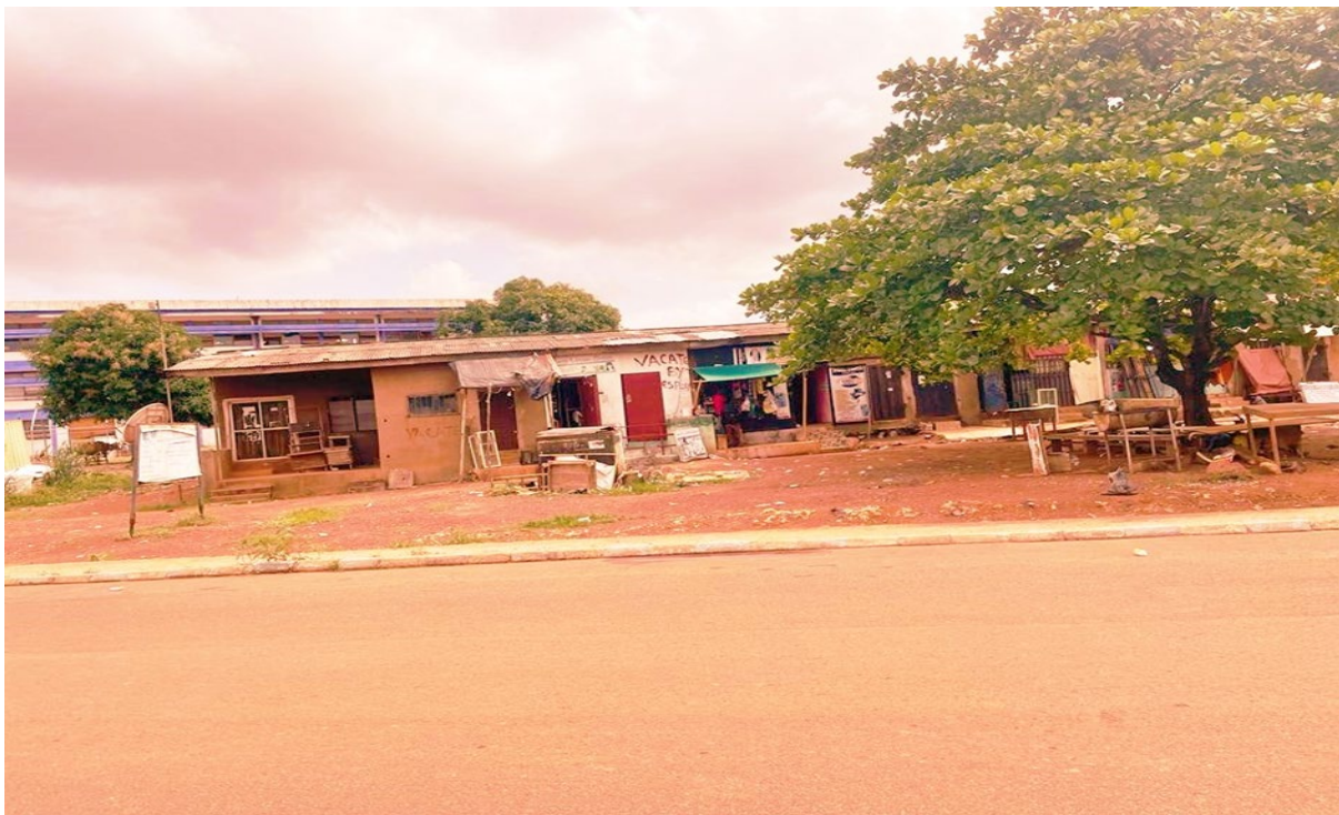
Plate 4: Picture showing the rear of the business premises behind the academic complex Drainage
