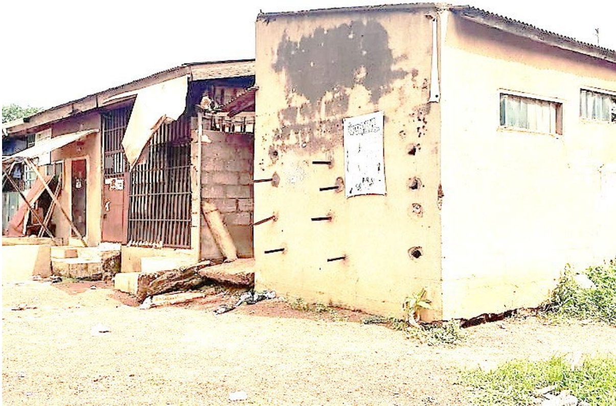
Plate 3: Picture showing the rear emergency exit in one of the prototypes in use
